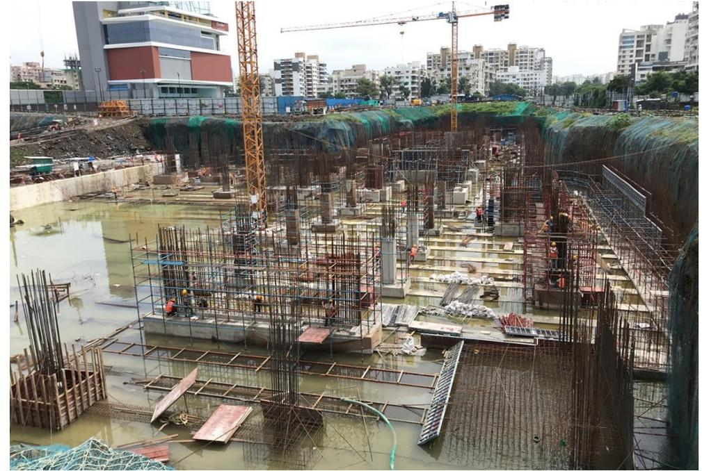
Excavation is complete, foundation & retaining wall work is in progress
