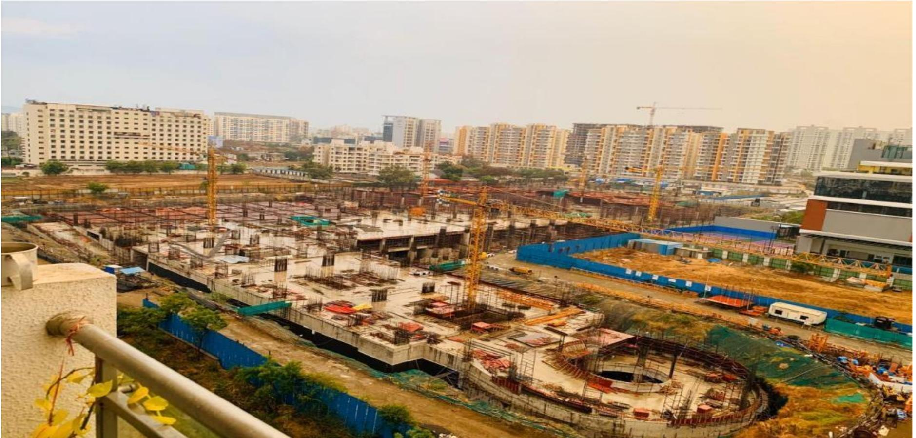
Foundation work is complete, Lower ground Floor Slab in progress
